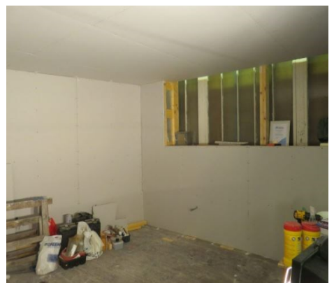
Pictured (top to bottom): CMS today with the plasterboard up on the walls and ceilings; the before and after of the log burner installation; insulation completed; and the plasterboard project is complete
