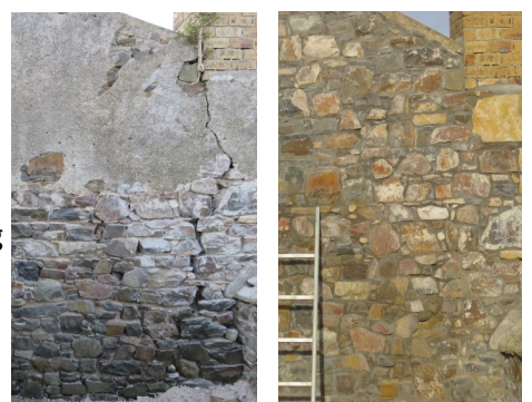
Pictured (top to bottom): building the internal walls and installing electrics; Stan Slater (pictured on the right) with his fellow Shedders before lockdown; the Shed space before the refurb began; and the pointing repair of the outside wall
